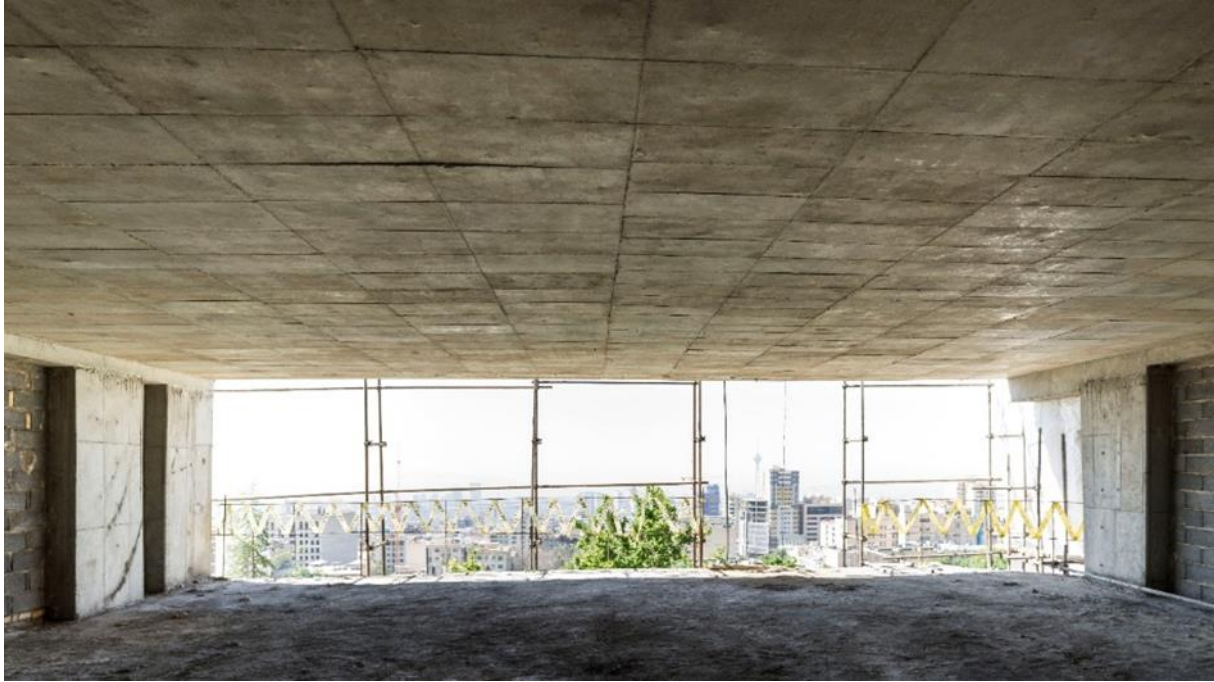
Figure 5.1. Floor made of Contruss voided slab
