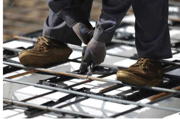
Figure 5.12. Contruss system construction
