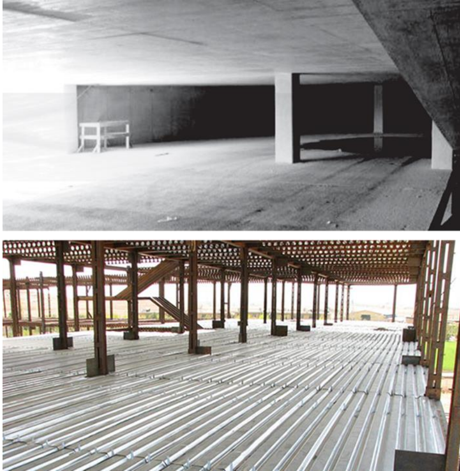
Figure 5.19. Contruss system compared to metal deck
