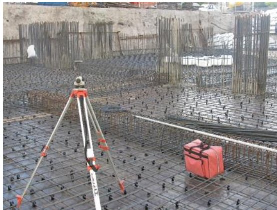
figure 3.2. Placement of lower rebar
