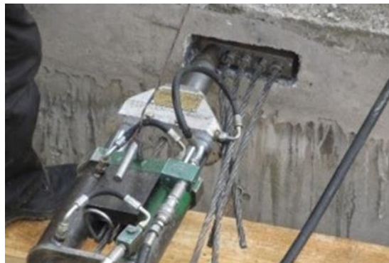
Figure 5.31. Post-tensioning the cables
