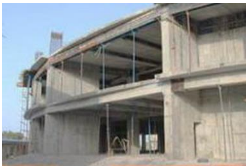
Figure 5.34. Construction with prestressed system
