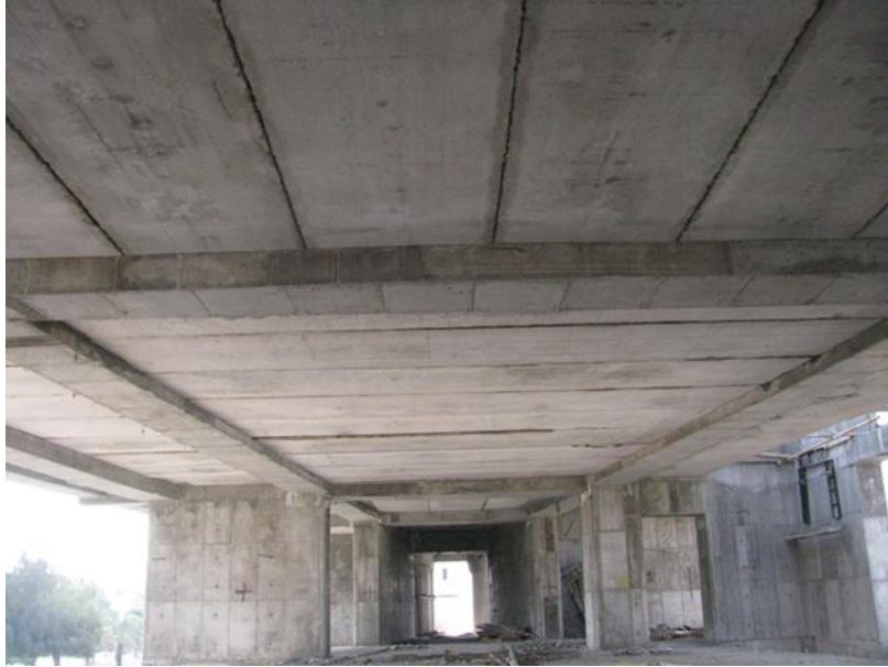
Figure 5.36. Floor constructed with prestressed system
