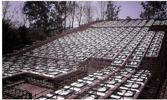
figure 3.4. Positioning the upper rebar
