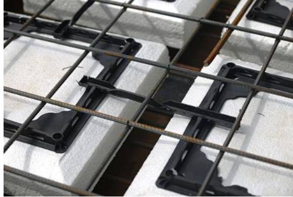
Figure 4.11. Providing clearance for rebar
