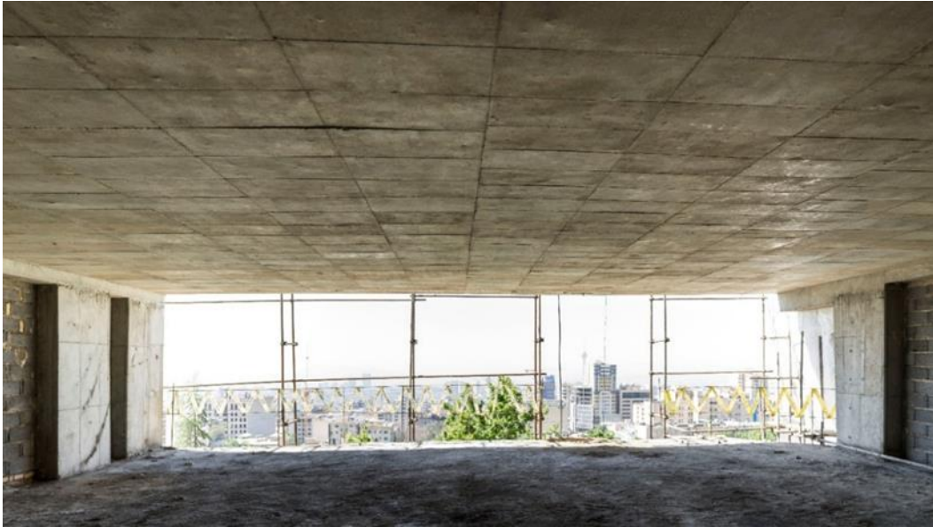
Figure 5.22. Floor made of Contruss voided slab
