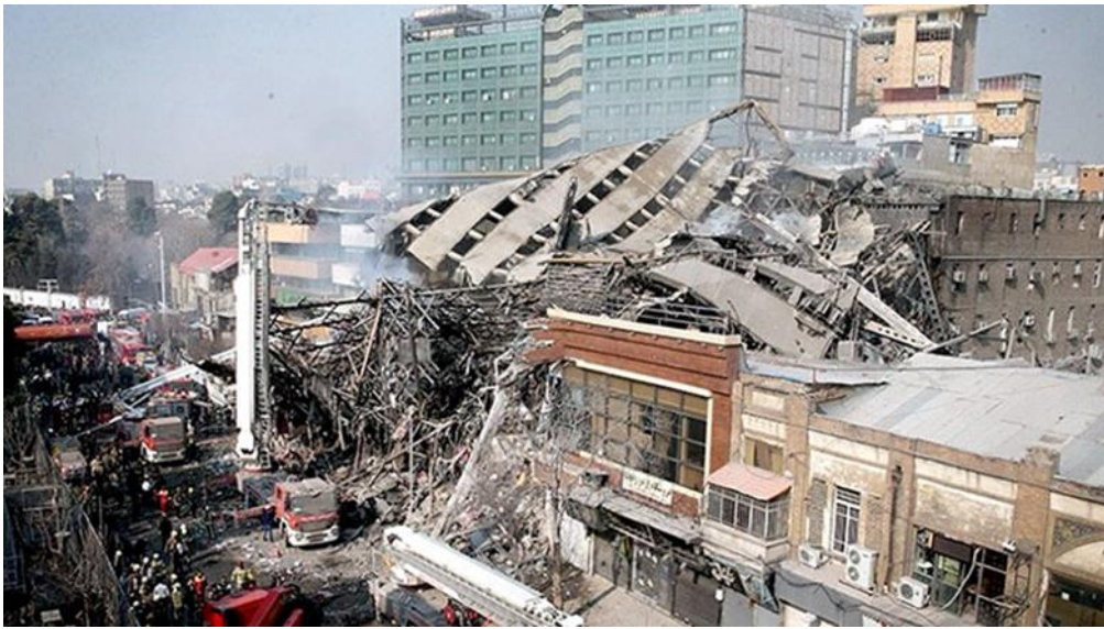
Figure 5.18. Metal deck collapse because of fire
