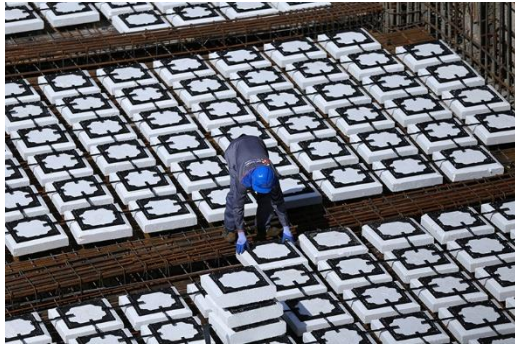
Figure 5.32. positioning of Contruss fillers
