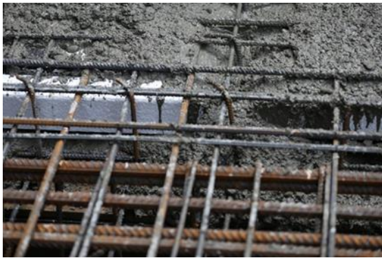
Figure 5.6. Contruss system construction
