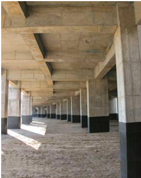
Figure 5.25. Beam and slab floor system
