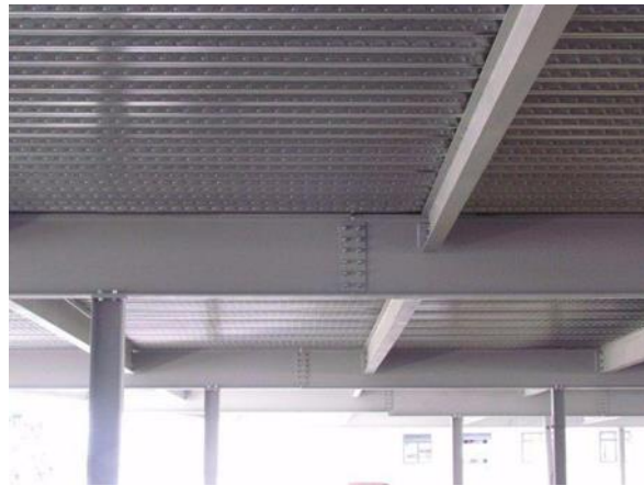
Figure 5.16. Thick girders in metal deck floors
