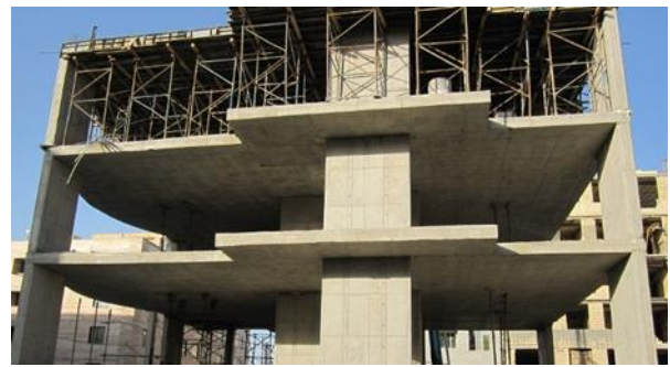
Figure 5.35. Construction with Contruss system
