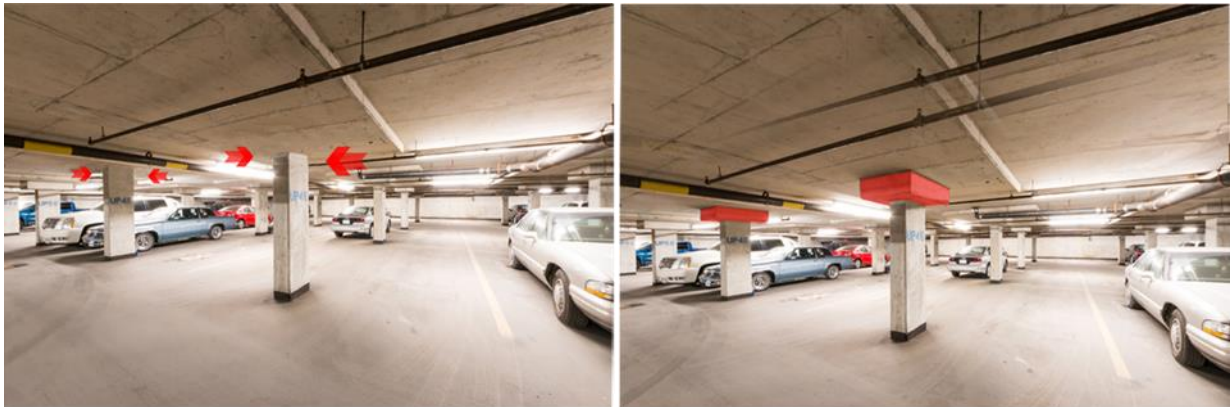
Figure 5.24. Aesthetic qualities after removing drop beams
