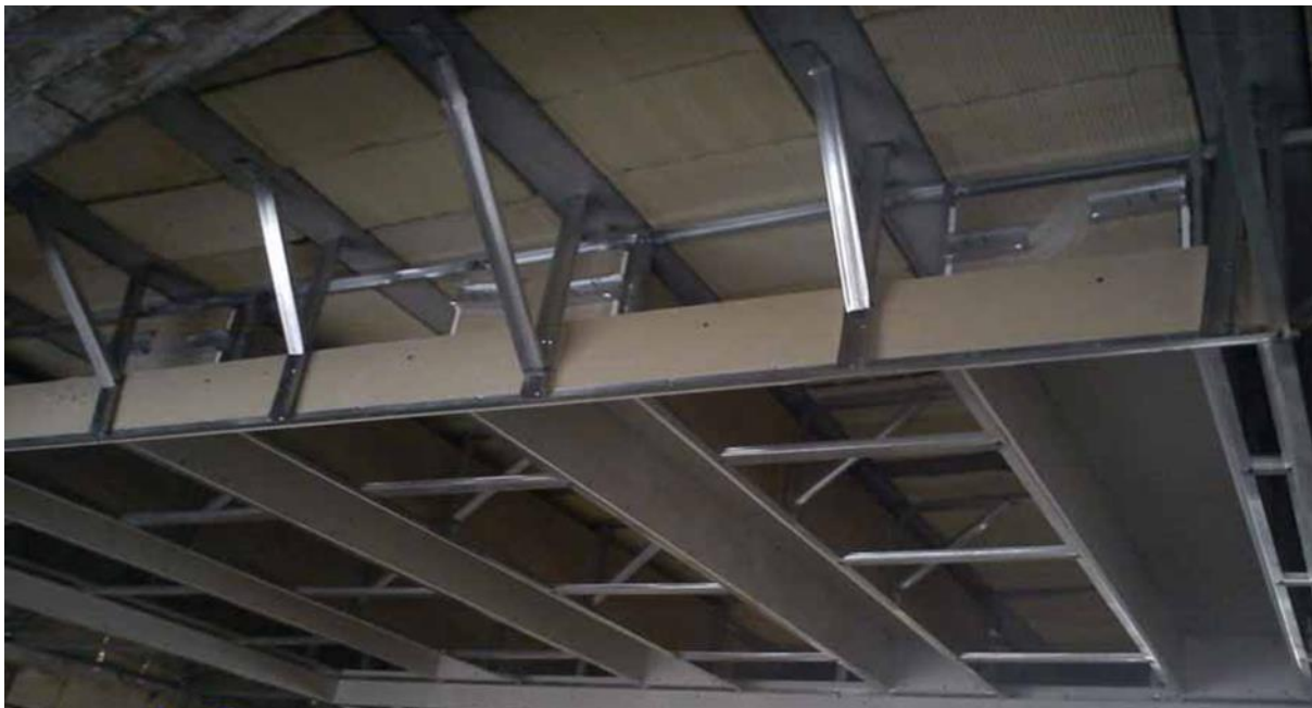
Figure 5.10. Dropped ceiling subframe
