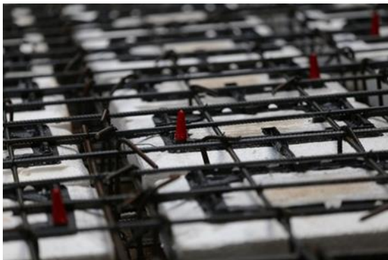
Figure 4.19. Indicators showing concrete thickness
