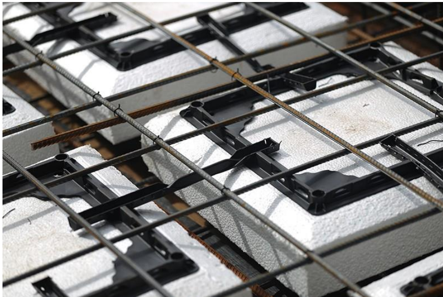
Figure 4.22. Positioning of upper rebar over belts
