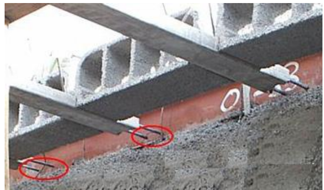
Figure 5.7. Rib and block construction
