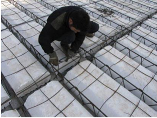
Figure 5.11. Rib and block slab construction
