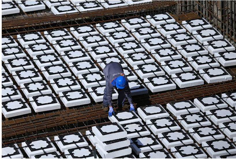
Figure 5.27. Positioning the Contruss fillers of voided slab
