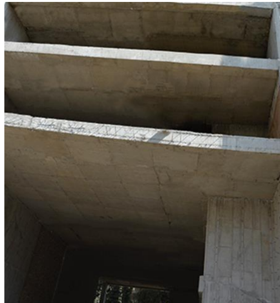
Figure 5.26. Contruss voided slab system
