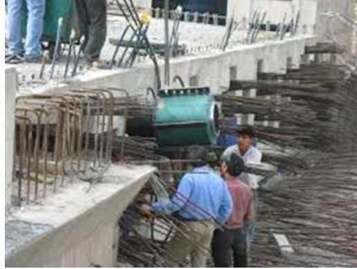
Figure 5.30. Pre-tensioning process
