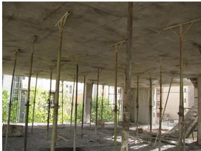
Figure 3.6. Removing the formwork
