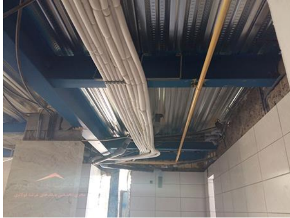
Figure 5.15. Passage of mechanical services below girders
