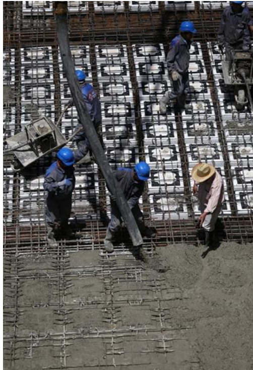
figure 4.21. Filler susceptibility during construction
