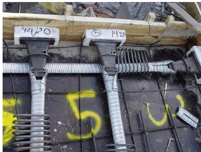
Figure 5.29. instruments of prestressed construction
