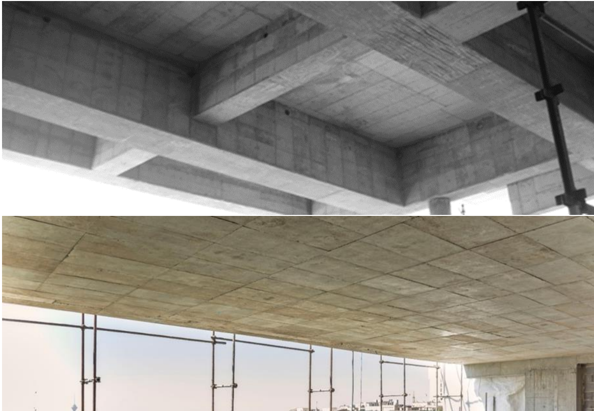
Figure 4.5. Creating a flat intrados floor
