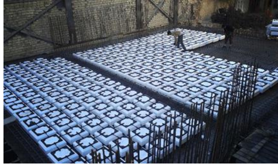
Figure 3.3. Placing the permanent fillers
