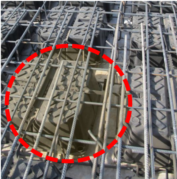
Inappropriate practical details for providing cover on U-boot filler
