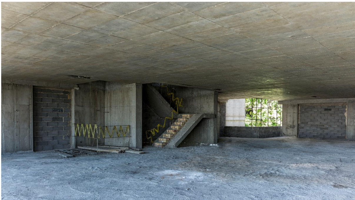
Voided slab created with Contruss filler
