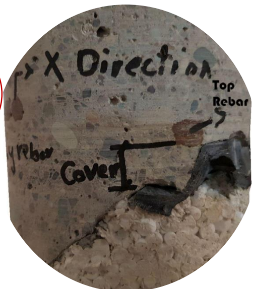
Tray on the Contruss filler provides appropriate cover
