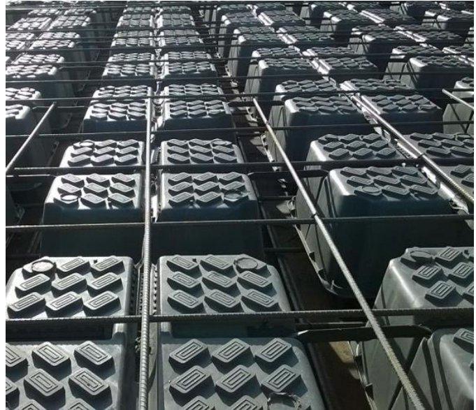
Inappropriate practical details for providing cover on U-boot filler
