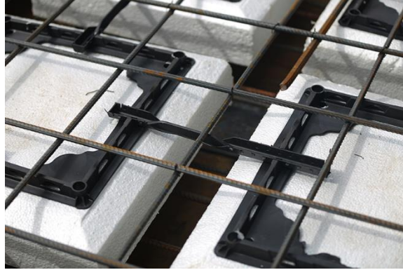
Trays to maintain reinforcement of Contruss filler
