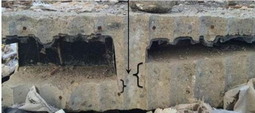
U-boot filler section- penetrating of the concrete inside the filler
