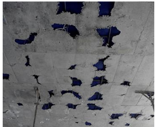
Ceiling created by U-boot system
