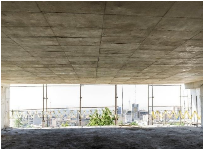
Ceiling created by Contruss system
