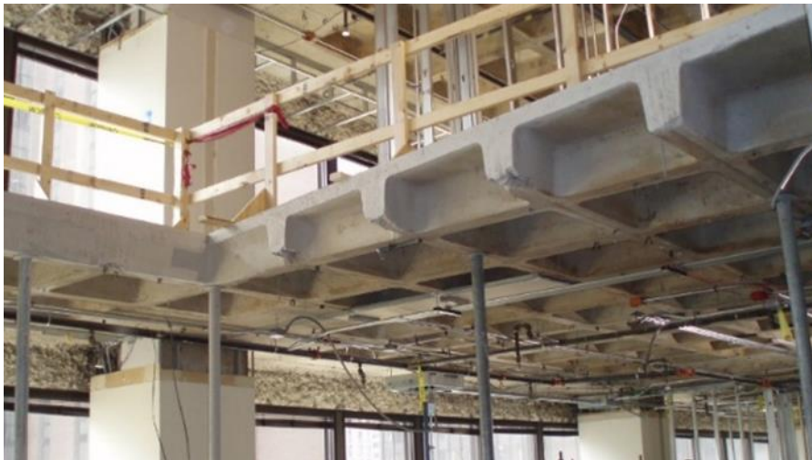
Figure 2.4. Waffle voided slab system
