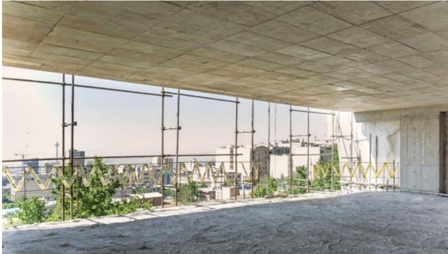
Figure 2.3. Contruss voided slab system
