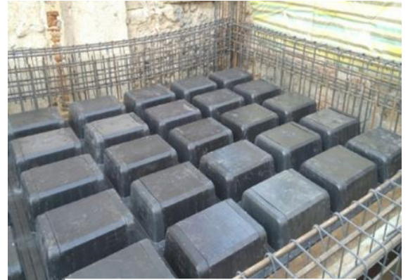
Figure 2.1. Waffle slab formwork
