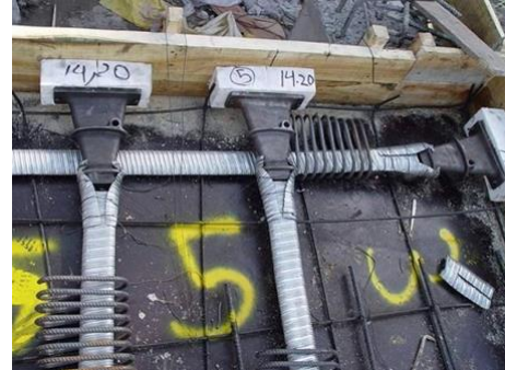
Figure 2.1. Positioning of strands
