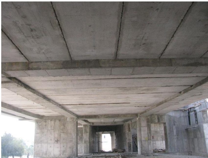
Figure 2.8. A prestressed ceiling system
