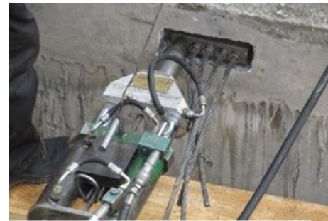
Figure 2.2. Releasing of strands
