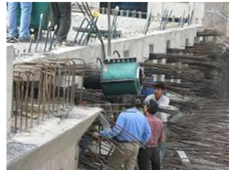
Figure 2.3. Prestressed system in bridge
