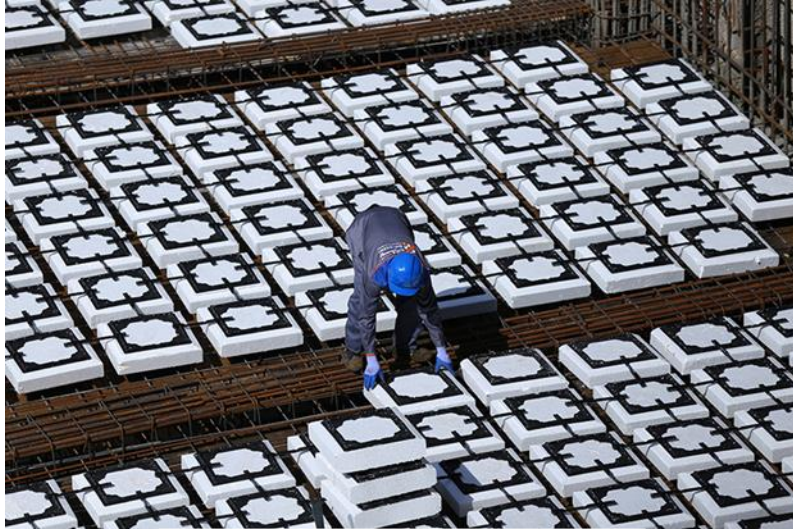
Figure 2.4. Contruss system installation
