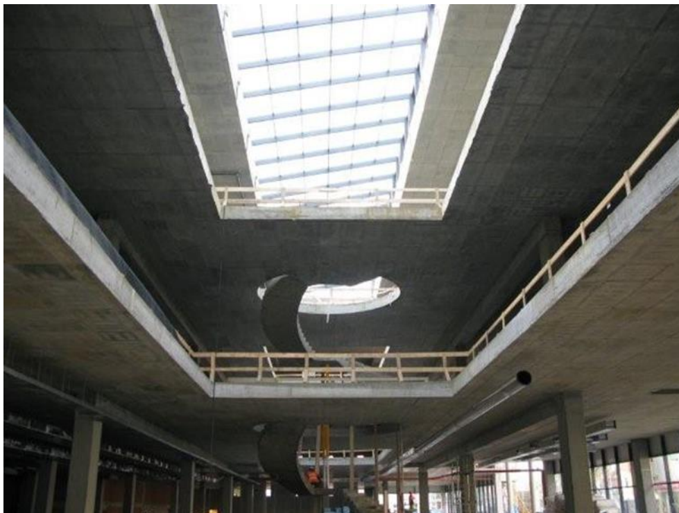
Figure 2.10. Created opening in the Contruss voided slab
