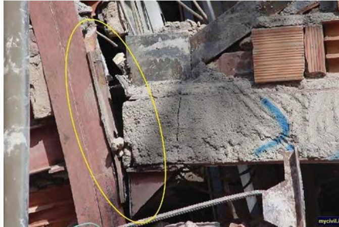
Figure 2.2. Welding fracture in steel structure
