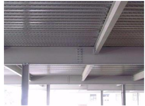
Figure 2.17. Large soffit in metal deck
