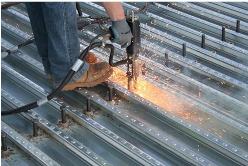
Figure 2.7. Installing stud shear in metal deck
