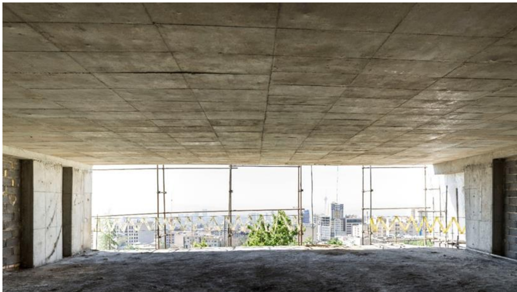
Figure 2.10. Large span provided in Contruss system
