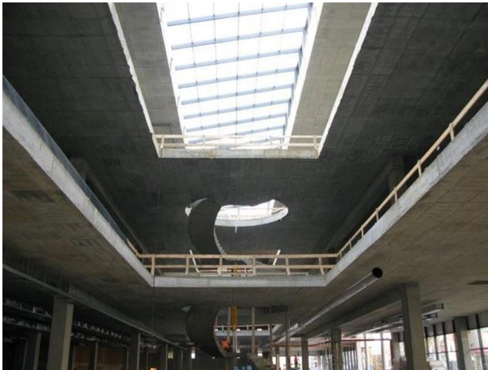
Figure 2.16. Ceiling constructed by Contruss voided slab
