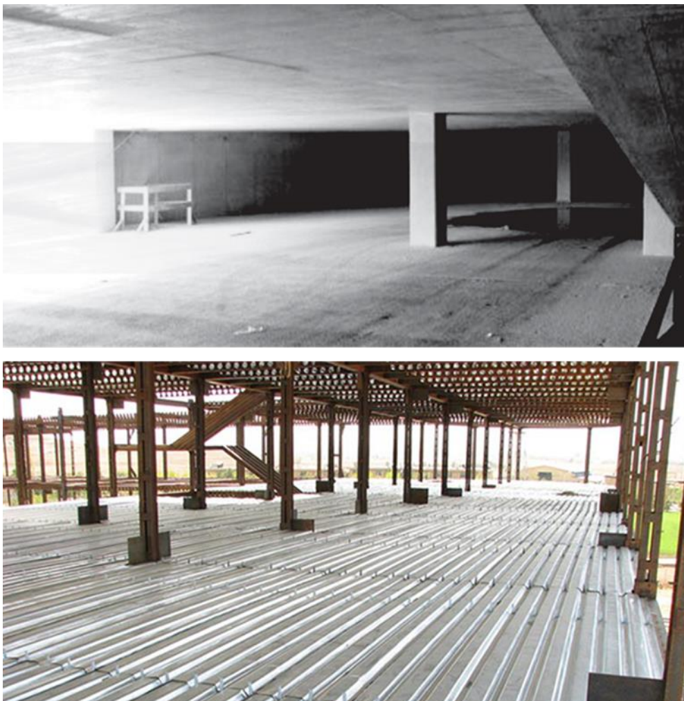
Figure 2.1. Comparison of Contruss with metal deck
