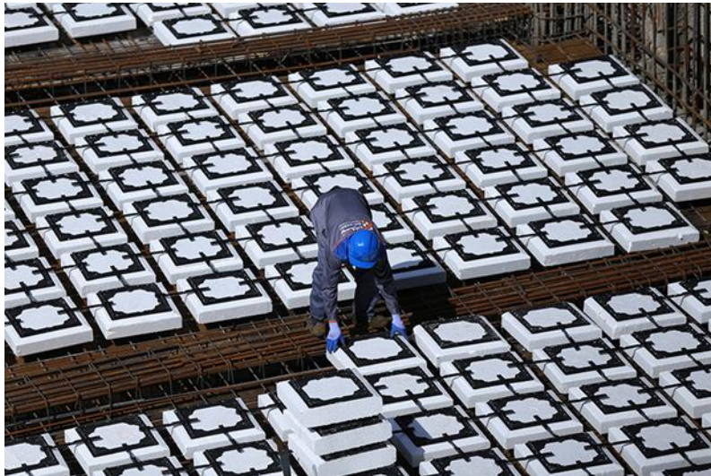
Figure 2.6. Installing the Contruss fillers on site
