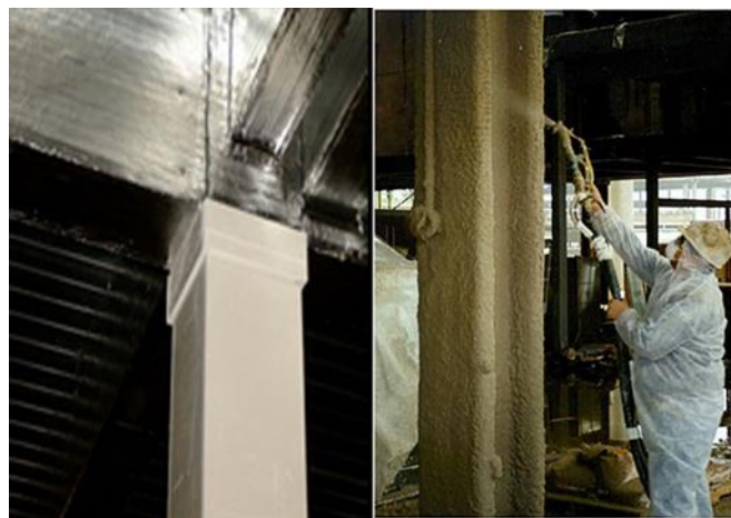
Figure 2.12. Thermal insulation in steel columns
