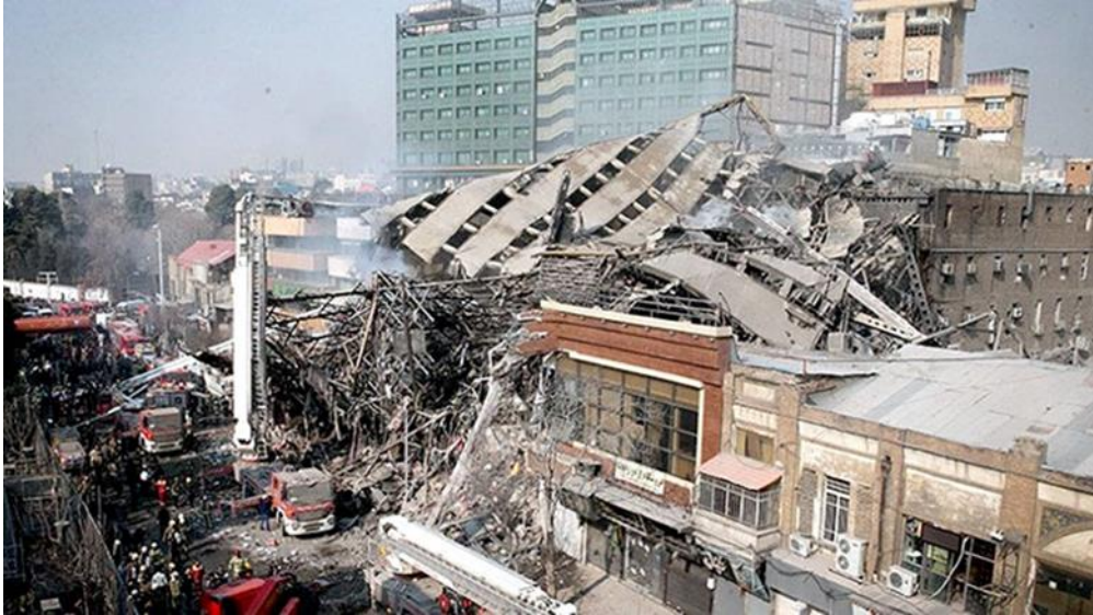
Figure 2.11. Collapsing of a steel structure in fire
