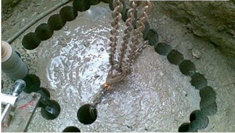
Figure 2.4. Creating opening in Contruss slab
