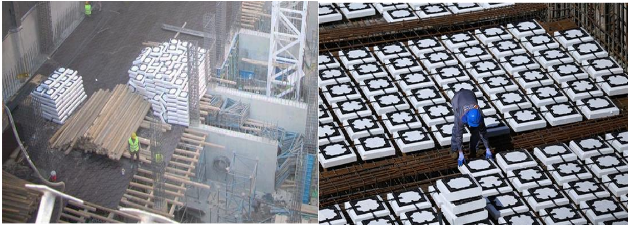
Figure 2.6. Installing Contruss voided slab
