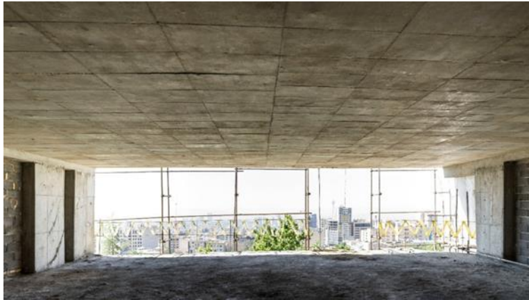
Figure 2.5. Simplified implementation of Contruss slab compared to slab-beam system
