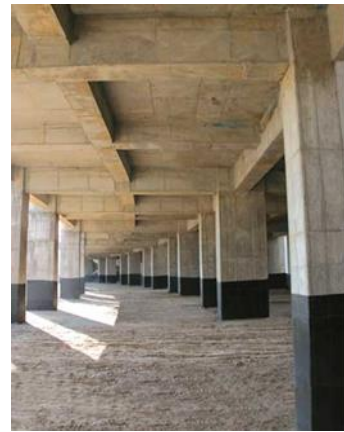
Figure 2.5. Simplified implementation of Contruss slab compared to slab-beam system
